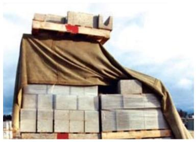
often comes from excessive wetting or saturation of recently built brickwork.
